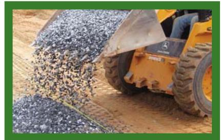
the lowest elevation of the wall. Level the prepared base with 6" of unreinforced concrete or well-compacted granular fill (gravel, road base or  $\frac{3}{4}$ " minus [13 – 20 mm] crushed stone). The leveling pad is typically 12" wider than the Mesa Unit, 6" in front and behind the Mesa Unit. Compact the well-graded stone to 95% Standard Proctor or greater.
